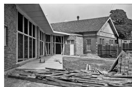
16 Harry Jensen Welfare Centre nearing completion, September 1958. The Abraham Mott Hall is in the background.
