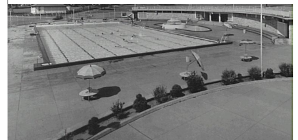
29 Swimming pool complex in Victoria Park. Source: CSA Unique ID A-00014927
