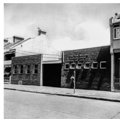
15 The Ron Williams Welfare Centre for the Aged in Kepos Street, Redfern. The open court within the building has since been roofed over.
