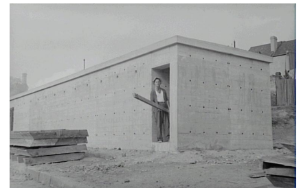
49 Concrete air raid shelter nearing completion.
