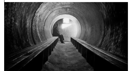
50 Cylindrical air raid shelter.
